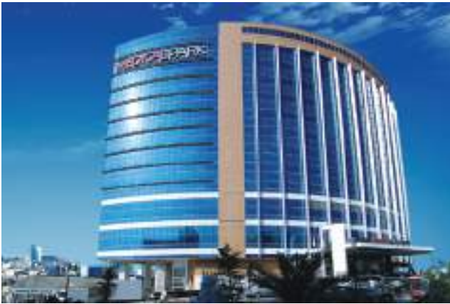
Medical Park Bahçelievler Hospital - İstanbul
